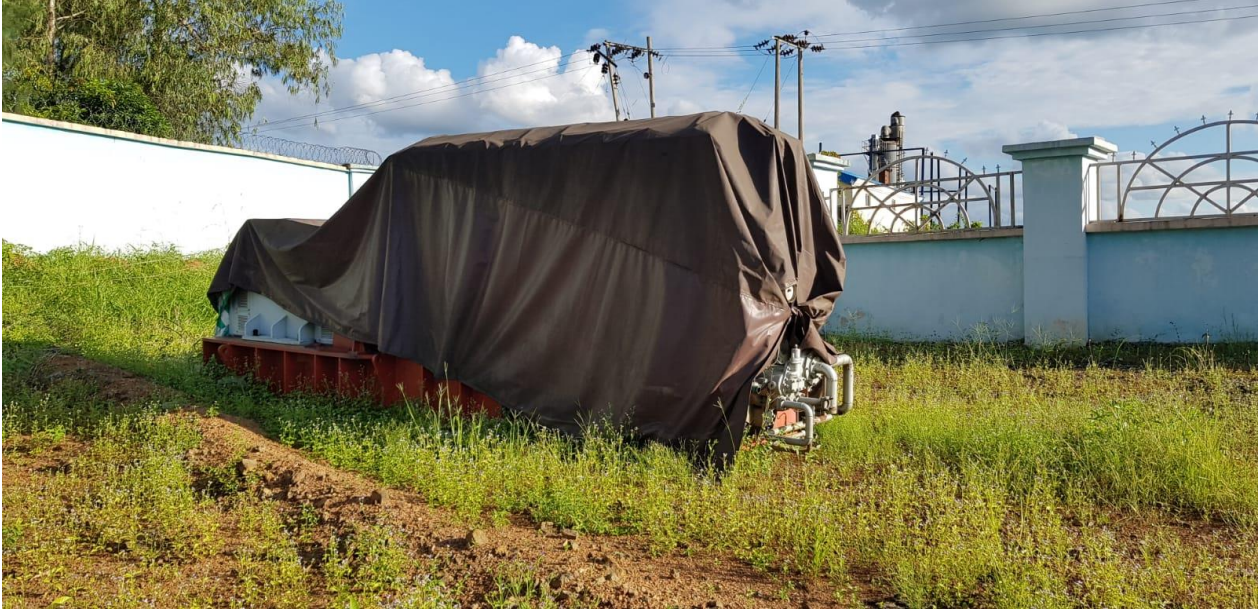
Condition of storage of 1 MW generator
